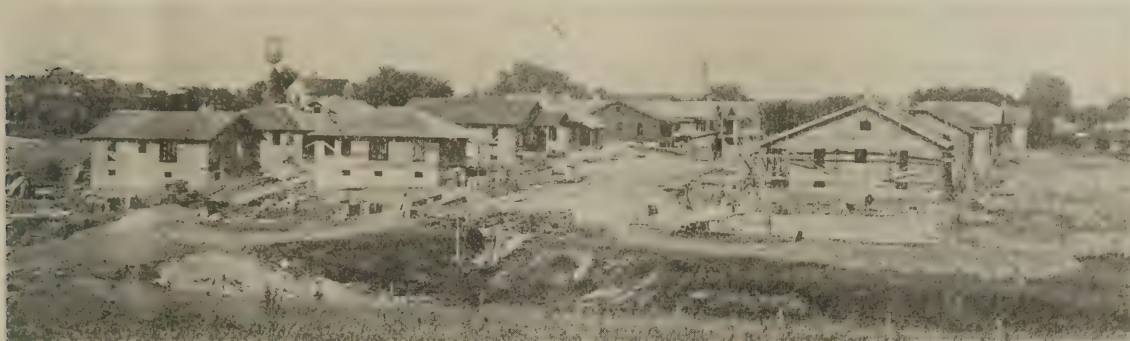
View showing progress of development
